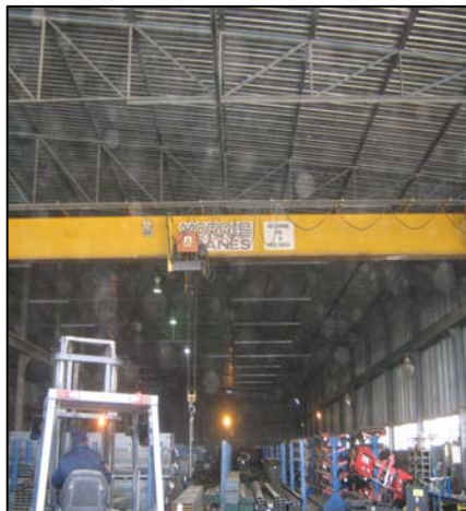
MAC STEEL OVERHEAD CRANE BUILDING
